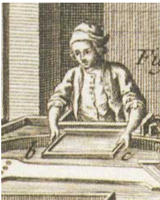
The vatman about to dip a paper mould into the vat. From the Encyclopédie of Diderot, 1751-1777. PD US accessed 8/23/17: http://www.wovepaper.co.uk/background.html
