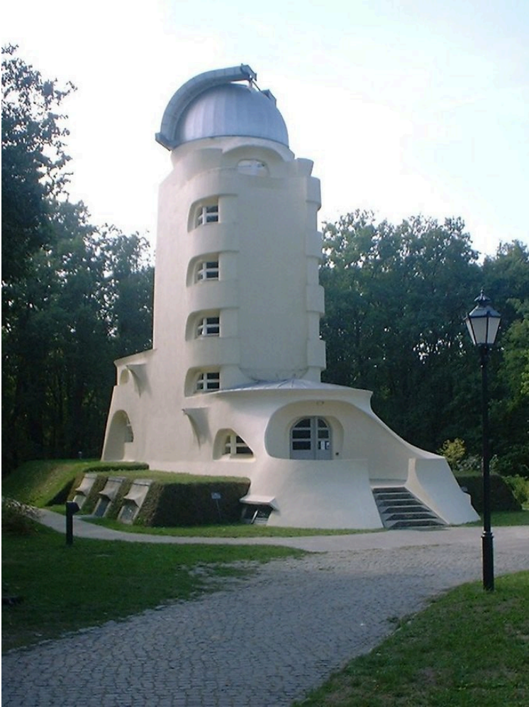
The Einstein Tower: In Mendelsohn's design, form and space are shaped in fluid concrete and devoid of applied ornament. Photo by Doris Antony, taken Sept. 16, 2003, CC BY-SA 2.5
