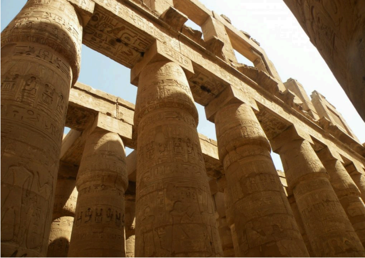
The Great Hypostyle Hall at Karnak, Luxor, Egypt. C. 19th Dynasty. Covers 54,000 sq. ft. An example of post and lintel construction. The columns are close together to support the weight of the lintel and the roof. CC PD, Free for personal and commercial use, No attribution required
