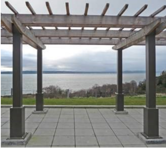
Post and lintel support in contemporary use; Image by Chris Gildow, Used with Permission
