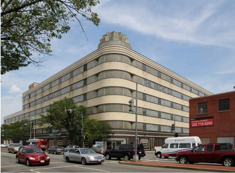
Hecht Company Warehouse: The Hecht Company Warehouse (Washington, D.C.) is a Streamline Moderne style building. The building uses glass block extensively, culminating in a twelve-pointed star-shaped cupola at the corner, which is illuminated at night. Black brick interspersed with glass block spells out The Hecht Co. at the fifth floor. Photo by Superbass taken July 12, 2012. CC BY-SA 3.0
