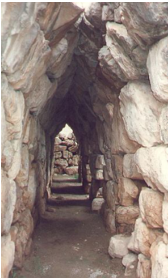
Corbeled vault, Tiryns: This photo shows the offsetting successive courses of stone at the springline of the walls so that they project towards the archway's center from each supporting side, until the courses meet at the apex of the archway. By User:Alexikoua, User:Panthera tigris tigris, TL User:Reedside - Ιστορία του Ελληνικού Έθνους, Εκδοτική Αθηνών , τ. Α' χάρτες σε σελ. 263-265, σελ. 290, 292-293 (επίσης [1], CC BY-SA 3.0
